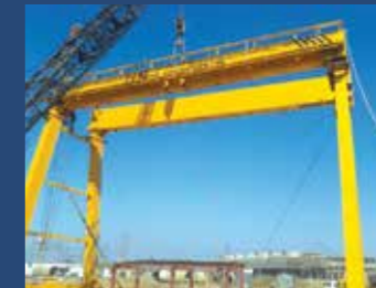
60T, Goliath Crane at Raigarh, Chhattisgarh Installation
