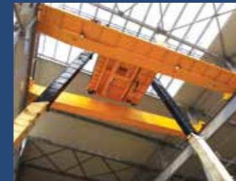
120T, DG EOT Crane Rajasthan, Erection & Installation
