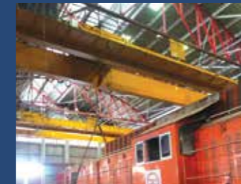
Refurbishment of old cranes
